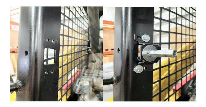
Step 2 & 3 - Locate your striker mount location, install, adjust and tighten your striker bolt and mount as illustrated above, secure using a 11 mm wrench and driver for this install.
